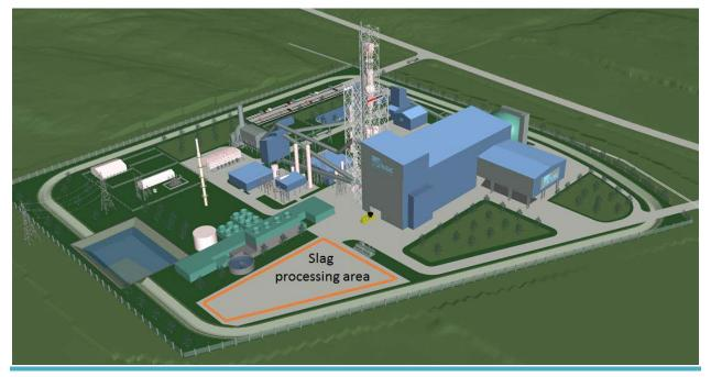
Figure 10.4-29.: location of the slag processing plant in the PURE FONTE LTÉE Layout
