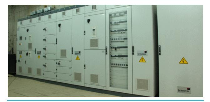
Figure 10.5-3.: Typical PLC Control Cabinet
