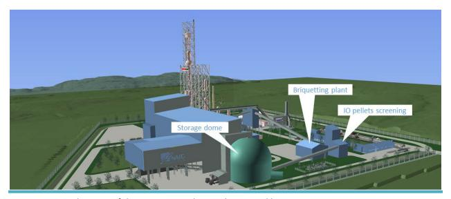
Figure 10.4-27.: location of the Briquetting plant in the general layout
